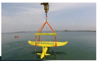
The first **0.5MW** utility-scale system of **Minesto**'s patented **Deep Green** technology has been commissioned at the Holyhead Deep site off the coast of North Wales, (October, 2018)
